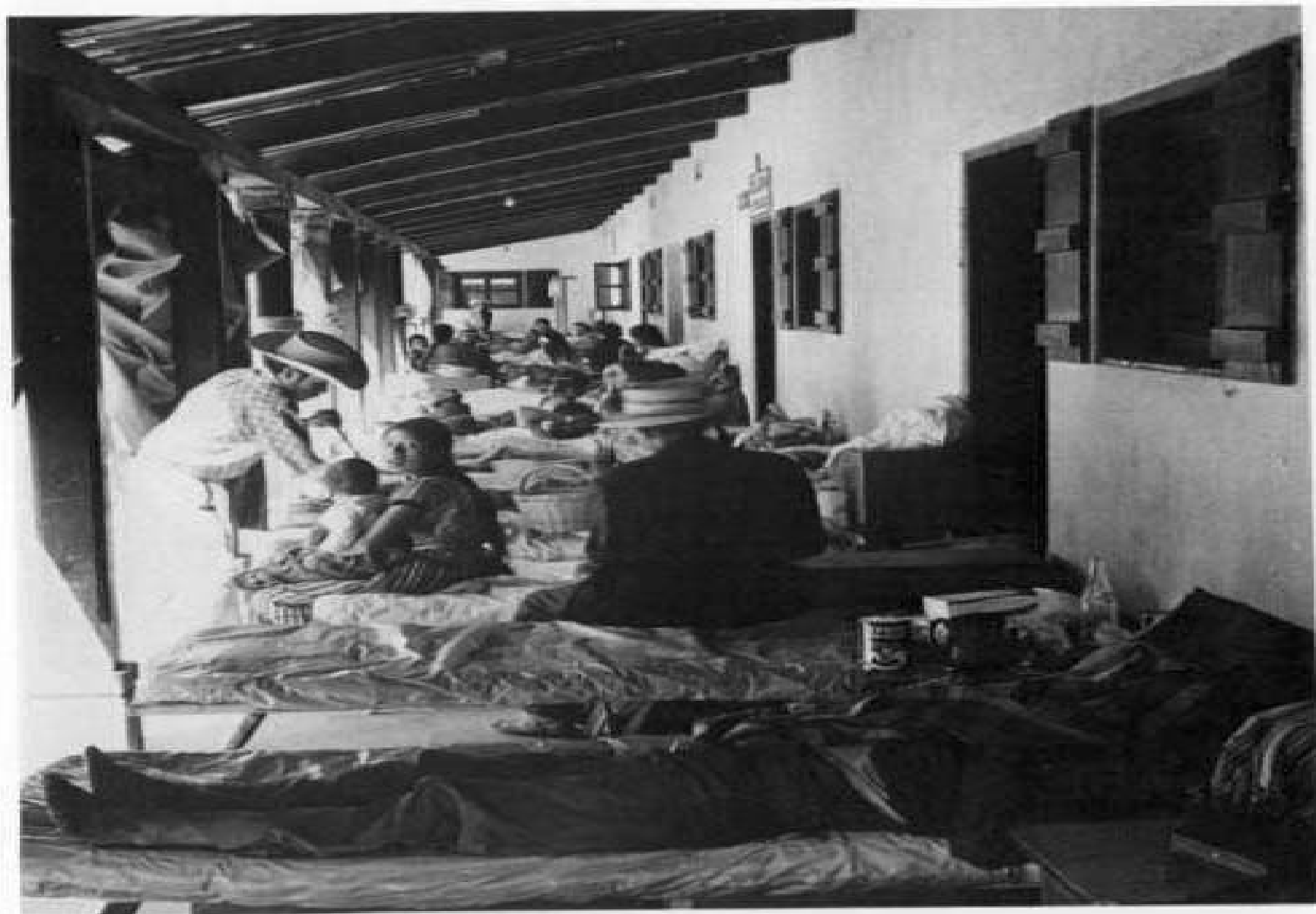
With beds inside and outside the one-story building, the hospital accommodates about sixty patients and their families who attend them
